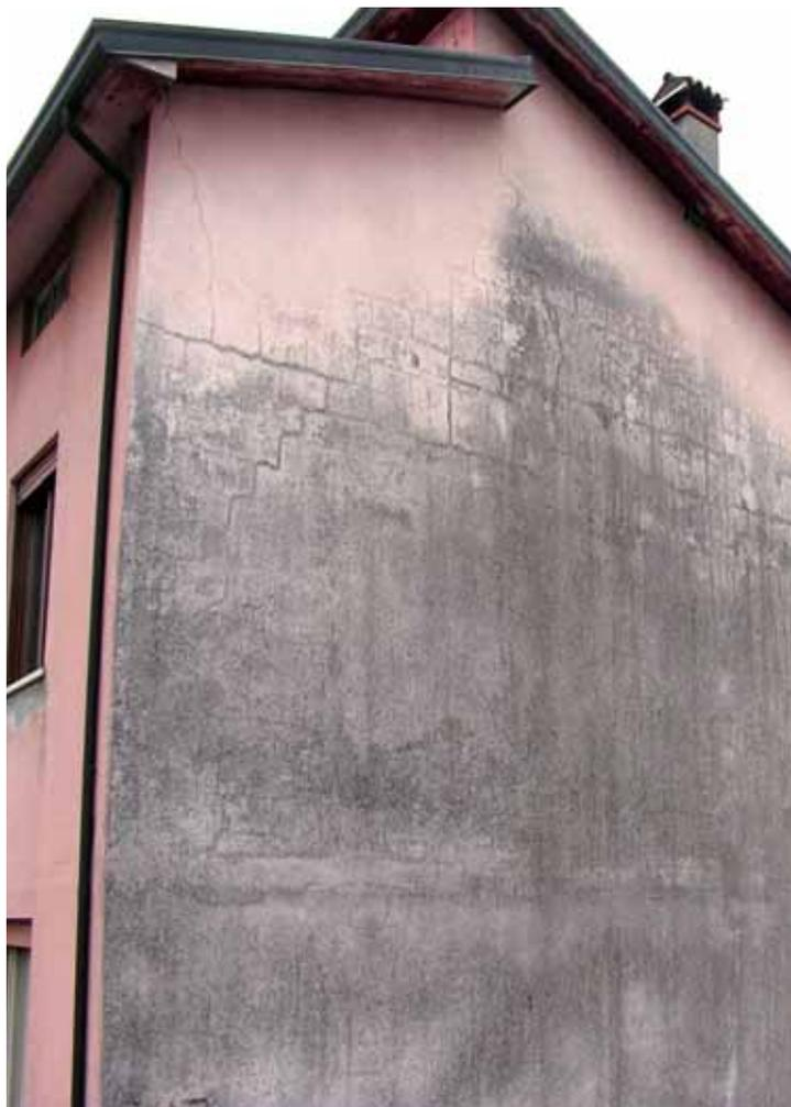
*The proliferation of micro-organisms, such as funguses and algae deriving from biological pollutants result in undesired effects such as patches & colour alterations. Sometimes the deterioration is such that it causes the progressive destruction of the existing paintwork & plastering.*
